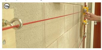
**11a.** Tension the system by holding the hexagon thimble whilst turning the switch eyebolt
